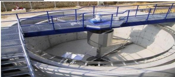
Sludge Thickening. Wastewater treatment plants commonly use thickening devices to increase the solids concentration at the end of a particular process step within the activated sludge process.
